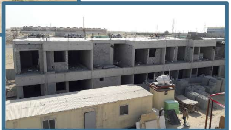
Block Works in Wing A and B
