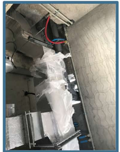
MEP- HVAC works on going
