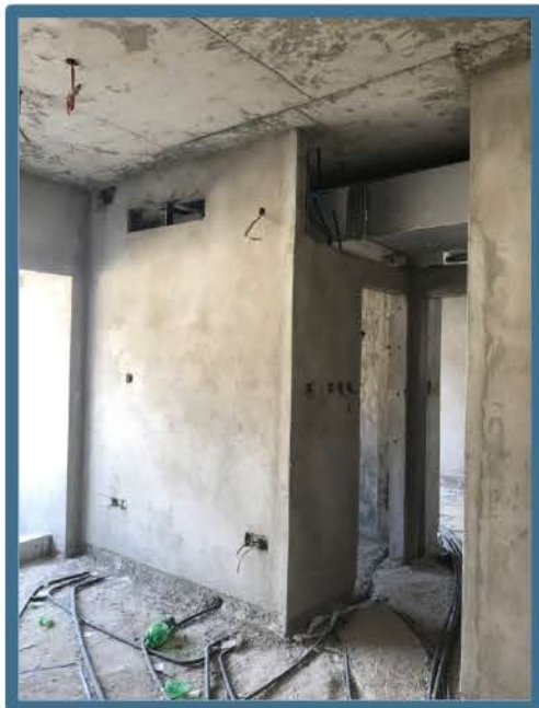
MEP- Electrical works on going
